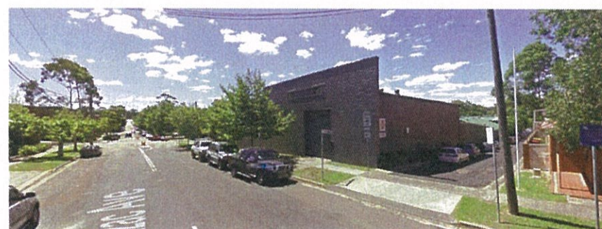
View from South East Corner
